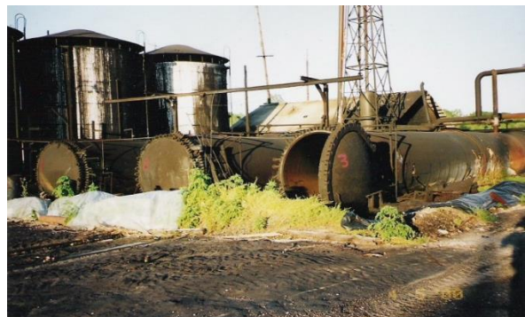
Abandoned Wood Treating Site
