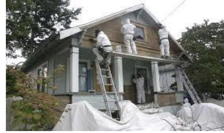
Lead-Based Paint Renovation Project
