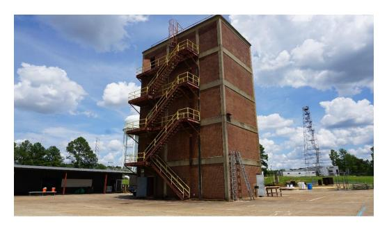
**Drill Tower:** The five-story drill tower provides opportunities for high-rise ladder, rope, and firefighting operations. In addition to this tower, there is a communications tower erected for training high angle rescue purposes.
